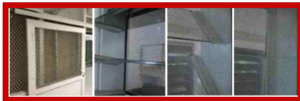
Figure 9: Doors and windows covered with wire mesh to prevent entry of dirt, dust, pests and birds
