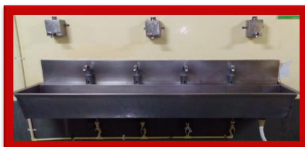
Fig 25 Foot Operated Hand Washing System
