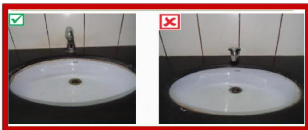
Figure 24: Touch free (hands free) taps at wash basins to avoid cross contamination
