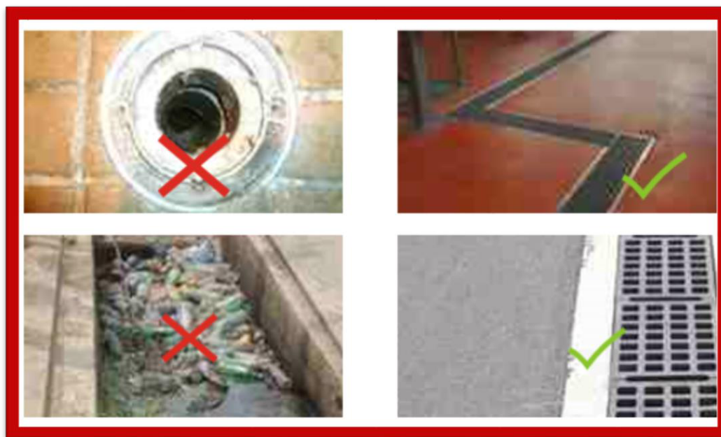
Figure10: Install covered drainage system inside the premises
