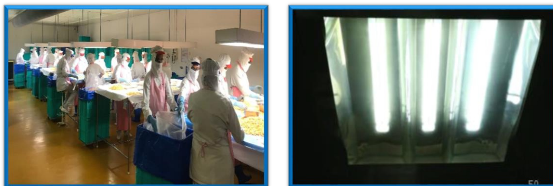
Fig 10- Adequate Intensity of light and covered fixtures
