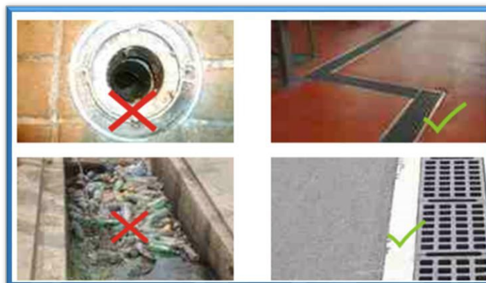
Fig 19- Keep no open drain inside the plant and Install covered drainage system inside the premises
