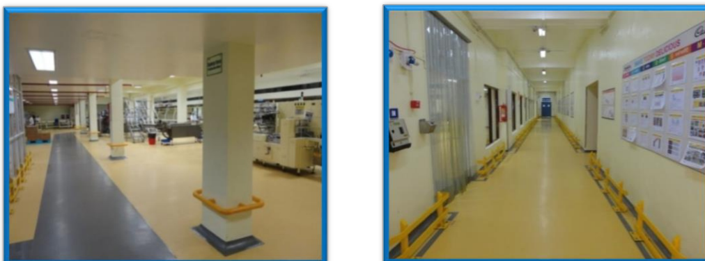
Fig 4- Wall and pillar guards used to avoid daily wear and tear of the surfaces
